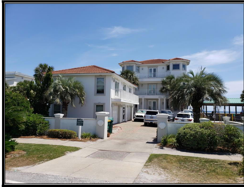
View of Subject Frontage along Scenic Highway 98 – Photo #1
