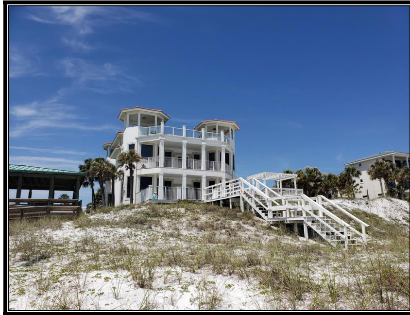
Side/Rear View of Main House & Beach Walkway (Facing Southwest Building Corner) – Photo #5
