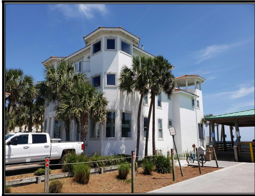
Front/Side View of Main House (Looking at Northwest Building Corner) – Photo #3
