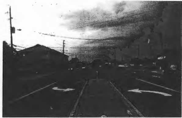
Existing US 98 looking West
