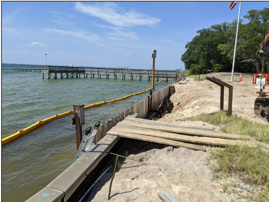
Figure 8. View of seawall installation, facing northeast.
