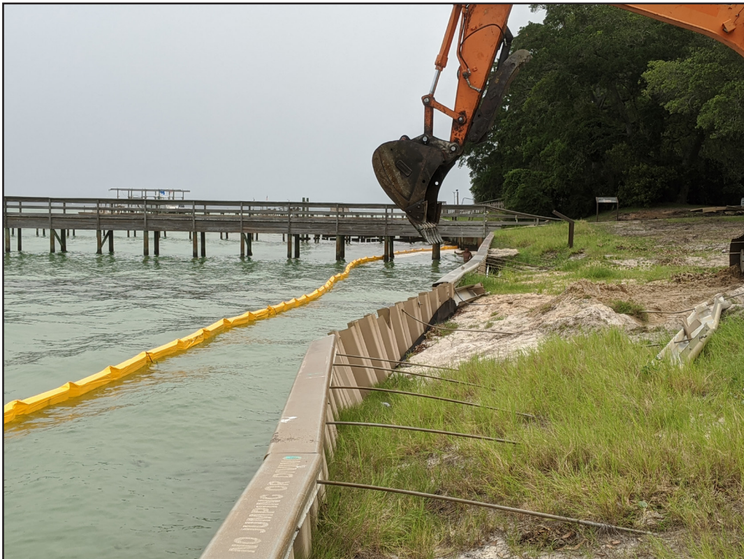
Figure 6. Removal of old seawall, facing northeast.
