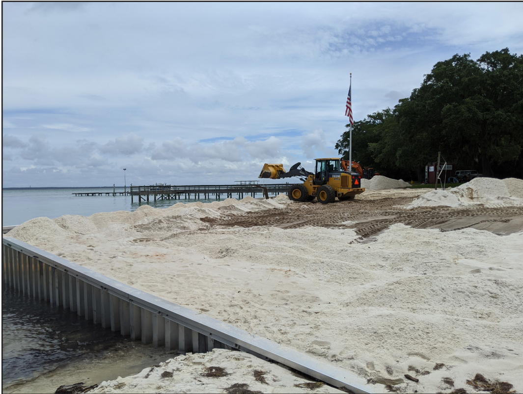
Figure 13. View of new white sand being spread, facing north.
