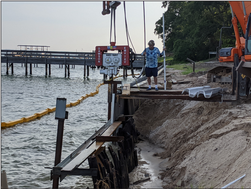
Figure 9. View of seawall installation, facing northeast.
