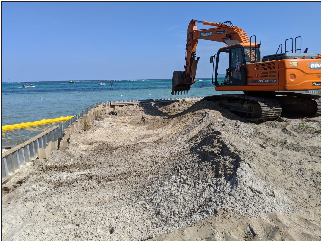
Figure 10. Prepping surface for anchor installation, facing northwest.
