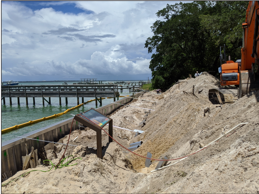
Figure 11. View of anchor installation, facing northeast.
