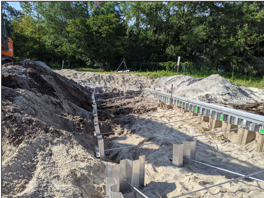
Figure 12. View of anchor installation, facing south.
