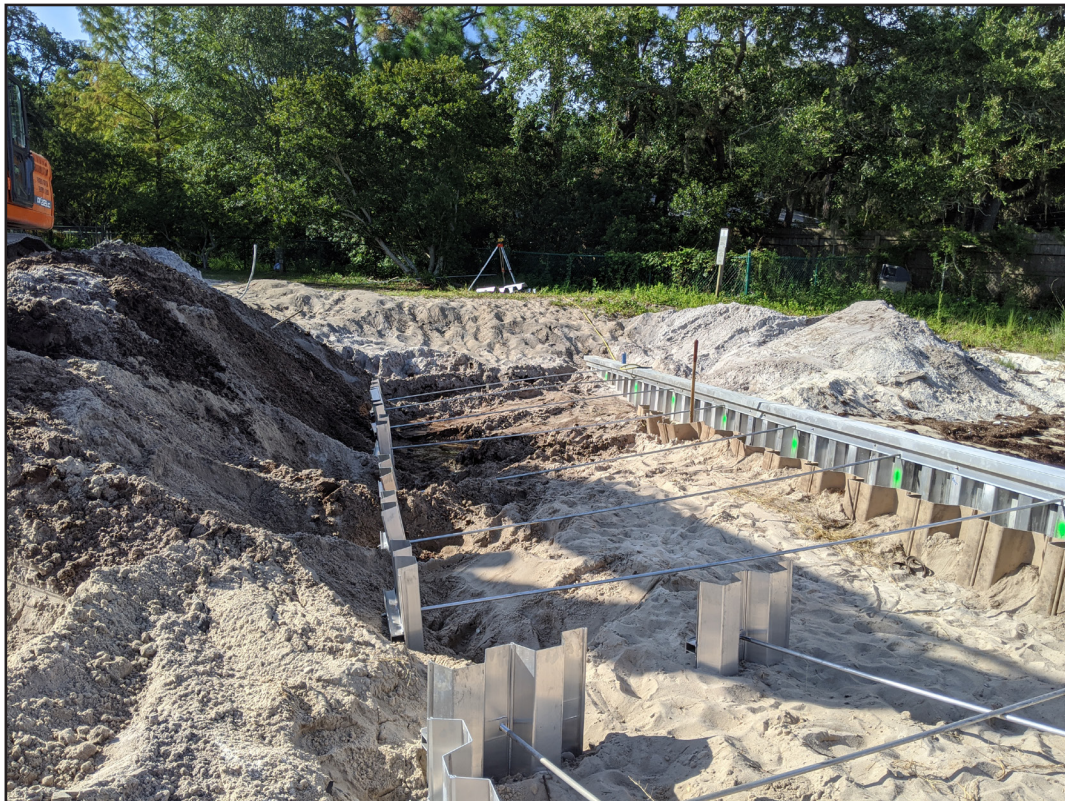
Figure 12. View of anchor installation, facing south.
