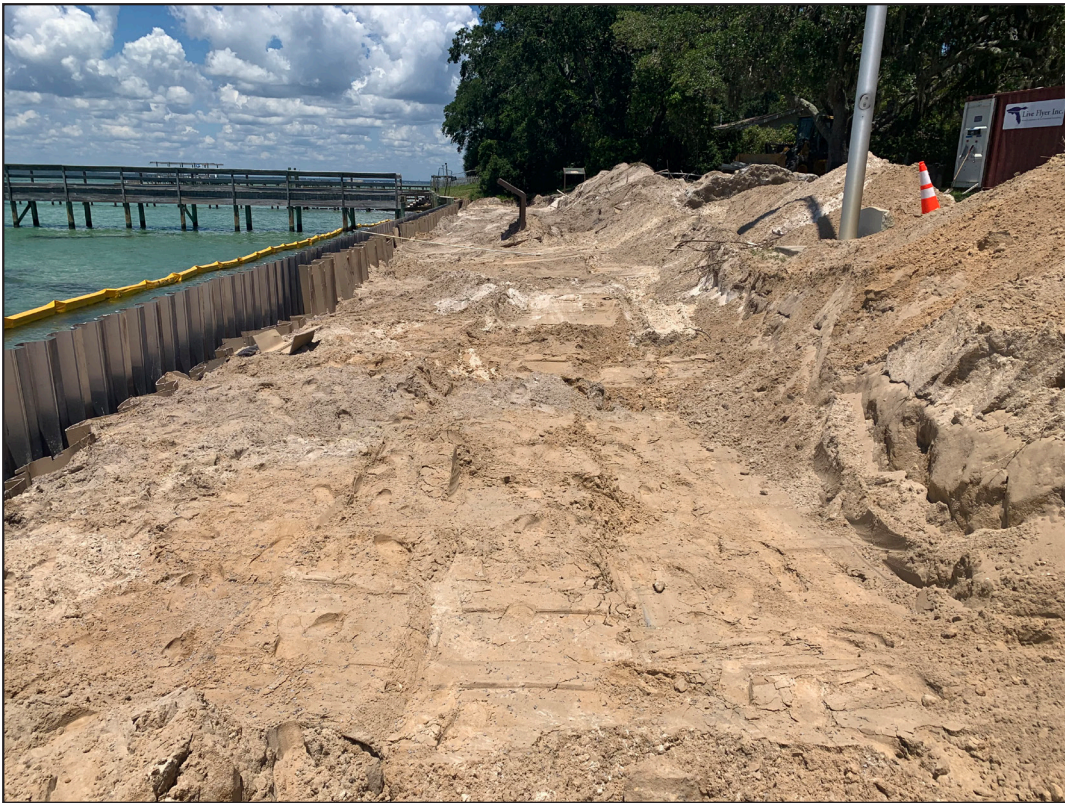
Figure 7. View of dirt pulled back from seawall during seawall construction, facing northeast.
