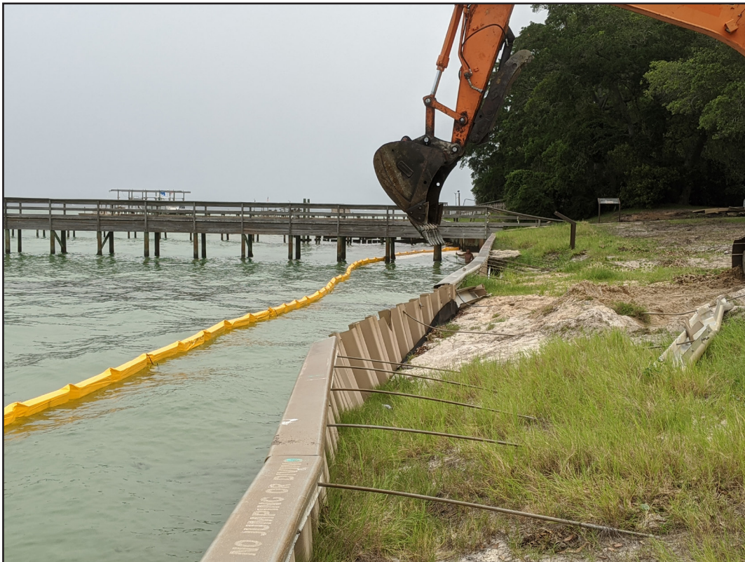
Figure 6. Removal of old seawall, facing northeast.
