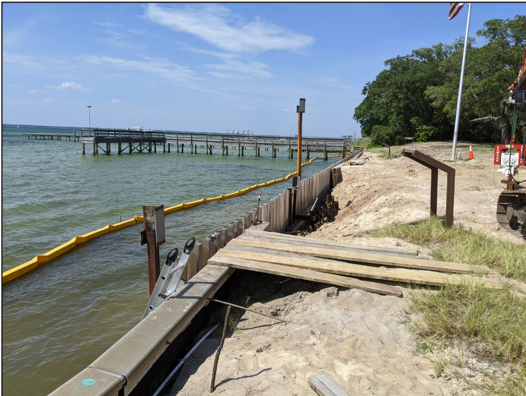
Figure 8. View of seawall installation, facing northeast.
