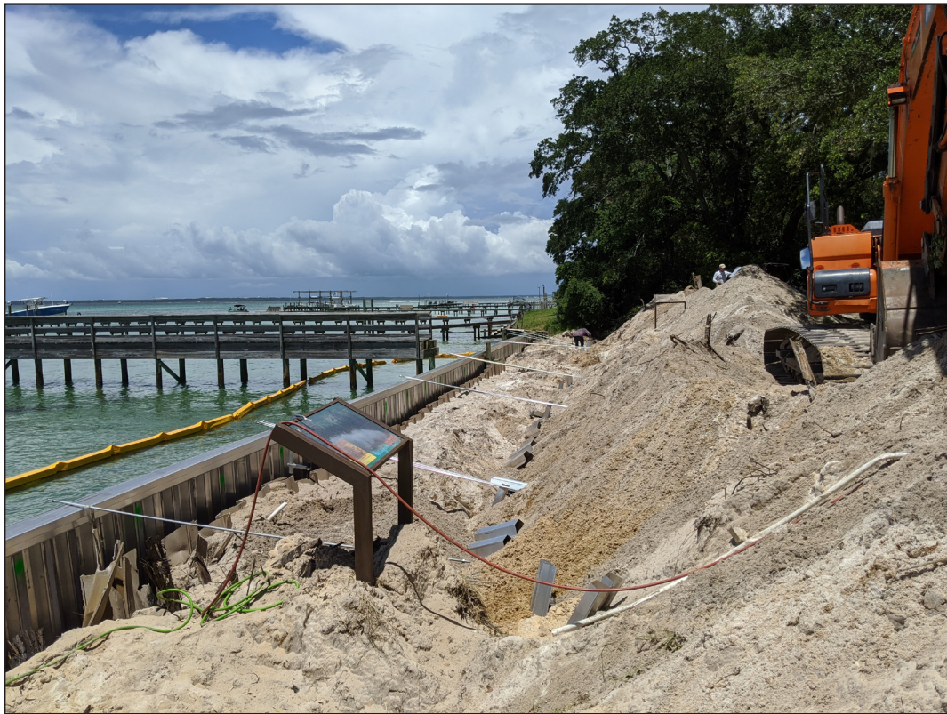
Figure 11. View of anchor installation, facing northeast.
