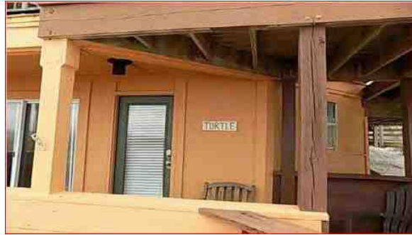
UNIT E LOCK OUT ON LOWER LEVEL
