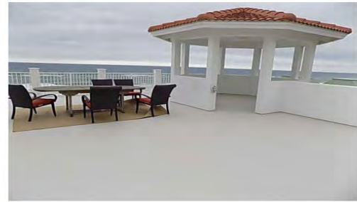
Top Floor Deck
