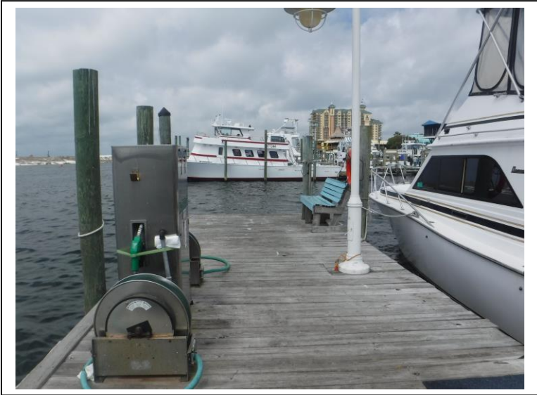
Photo 5: West end of terminal platform of East dock
