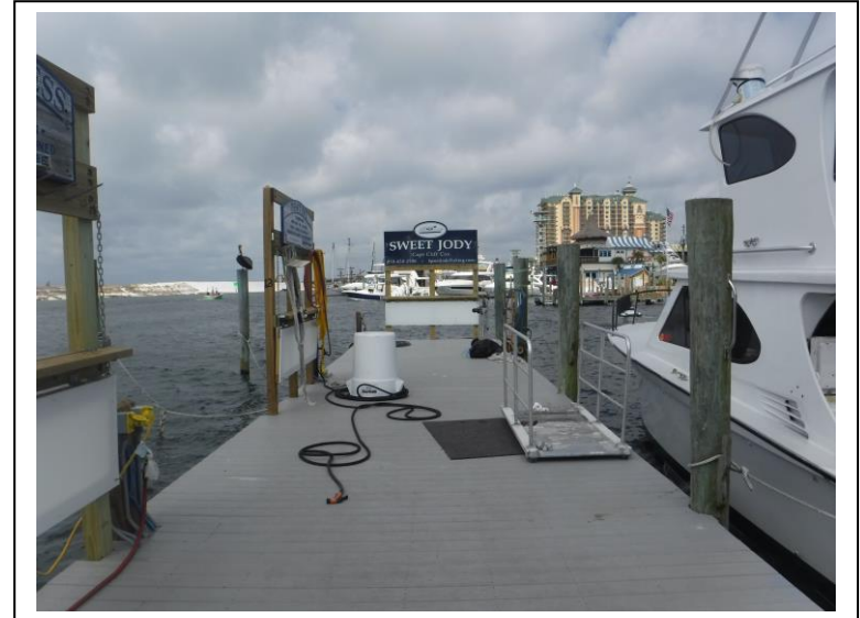
Photo 2: West end of terminal platform of West dock
