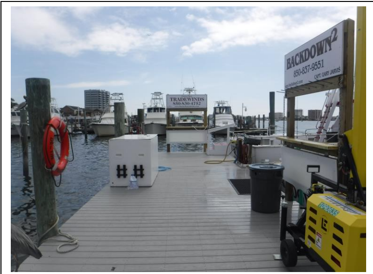
Photo 3: East end of terminal platform of West dock
