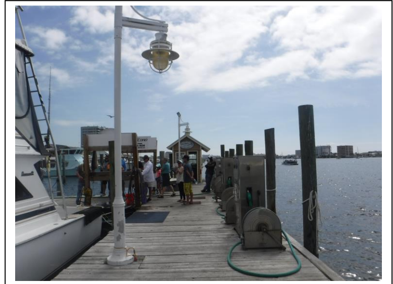
Photo 6: East end of terminal platform of East dock
