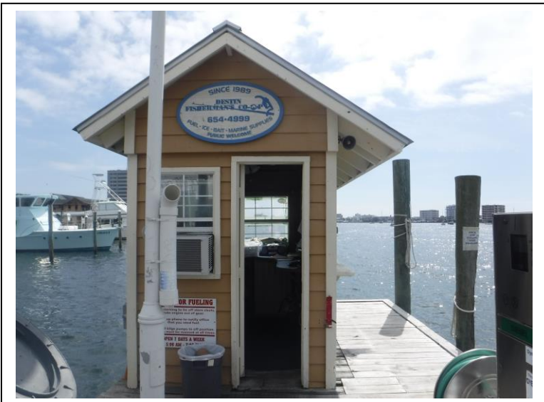
Photo 7: Shed located on East end of terminal platform of East dock.
