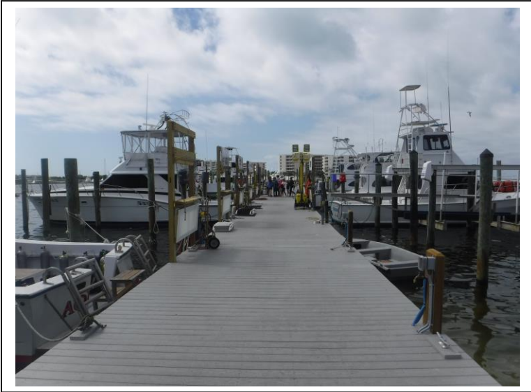
Photo 1: Waterward showing main access platform of West dock
