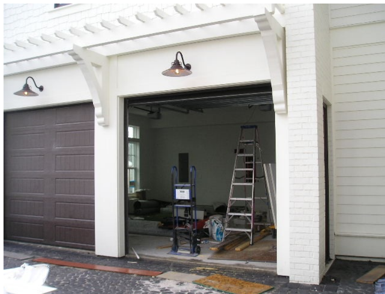
REAR OF SUBJECT
