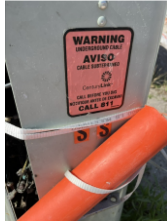
Telephone box (SS) Highway 98 Mapco (corner Of Guld Shore Dr. and Highway 98
