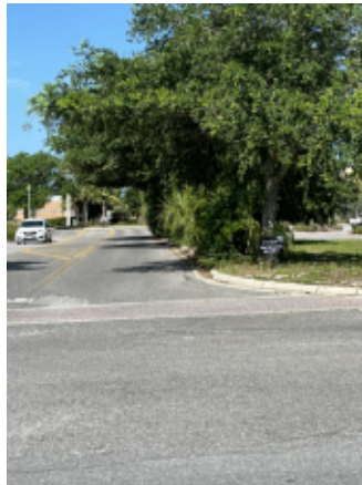
Growth over curbing Beside Walgreen's
