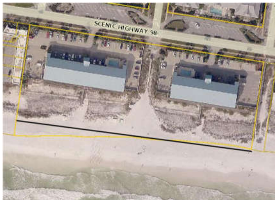
2: SAND FENCE INSTALLATION: 83 Sections over 740 ft. (Black Line)
