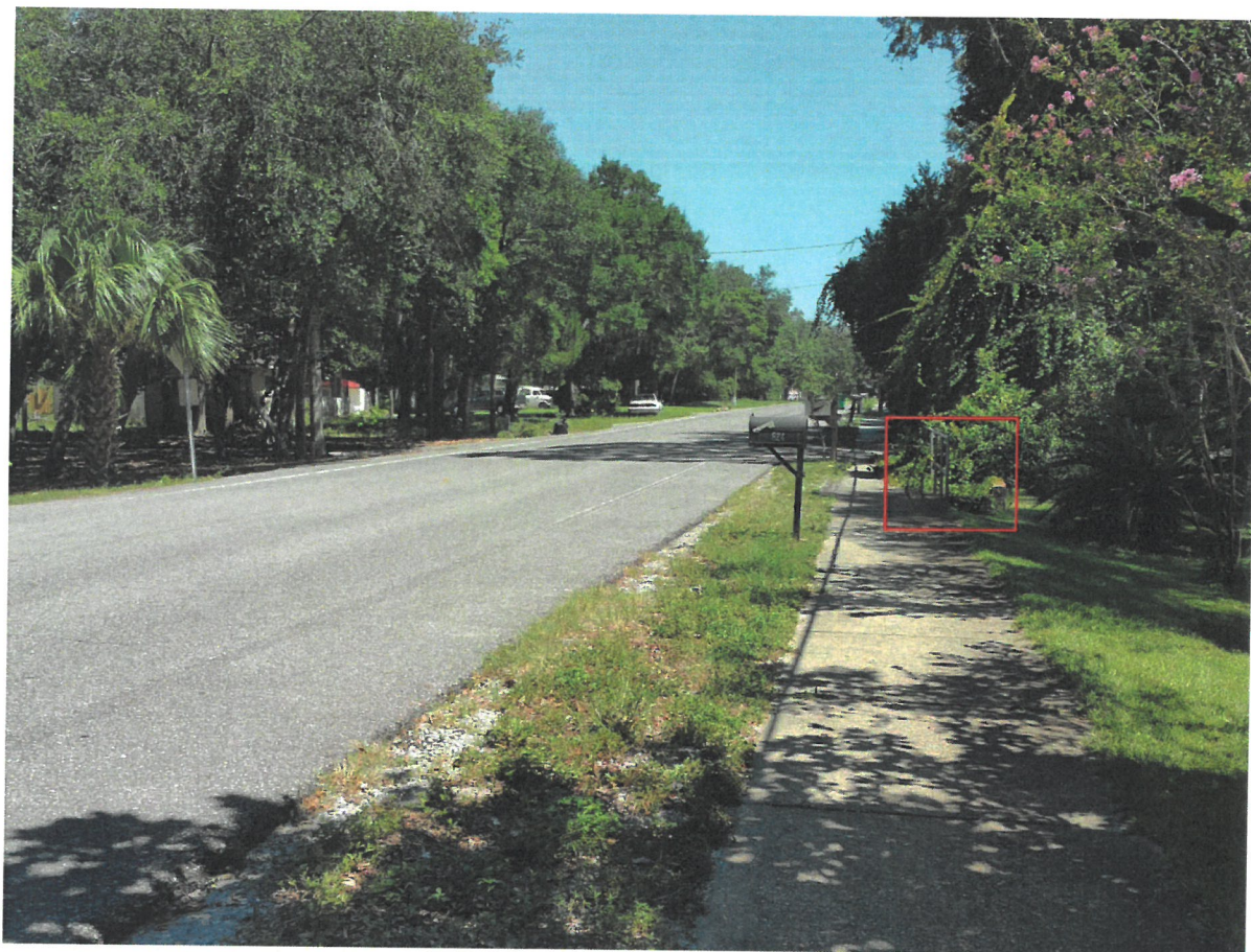
View of Cross St. (drainage shown in red box)
