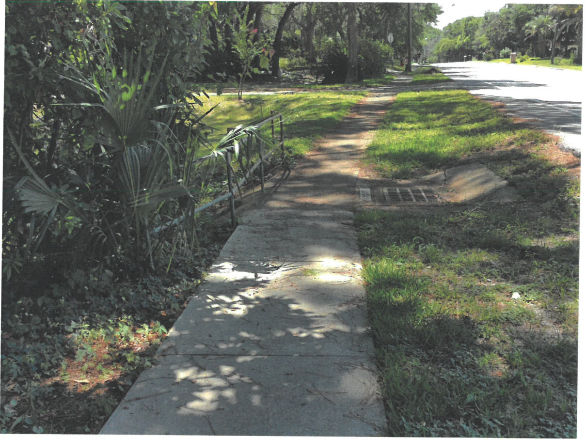
Upstream inlet and culvert structure along Calhoun Ave. discharging to outfall
