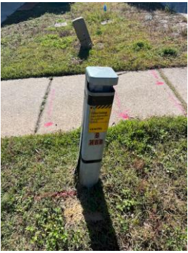
Telephone Box HBB6 3771 Misty Way
