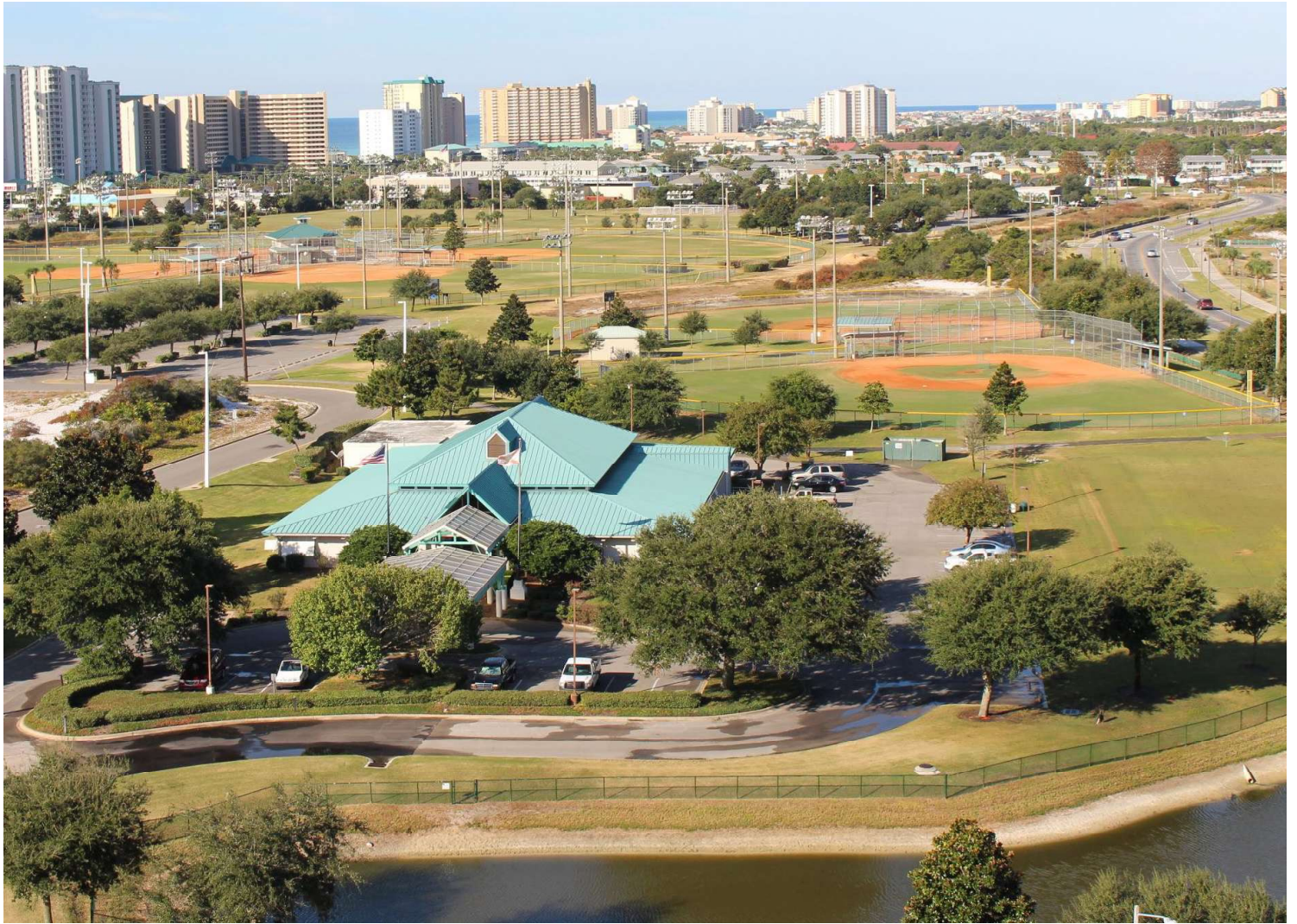
EXISTING CITY HALL
