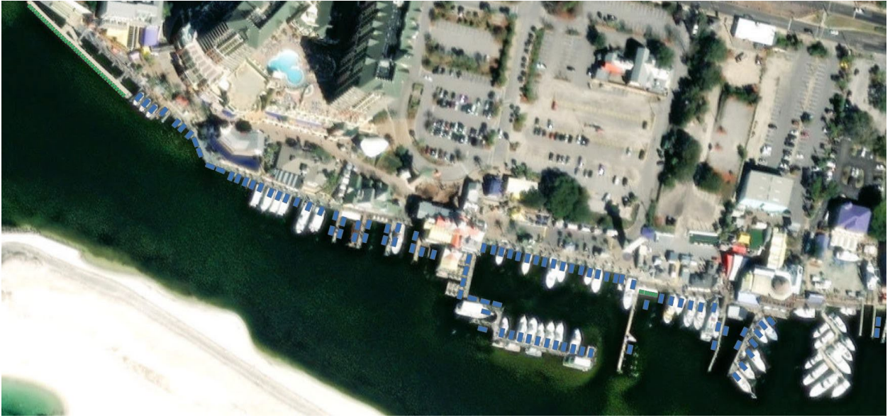
Figure 7: West side of GIS Slippage Capacity Count
