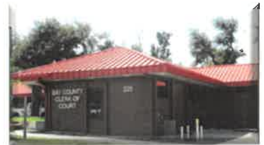
Bay Co. Board of Co. Commissioners Clerk of the Court Office Remodel* | Muni | Cost: $993,000 | Size: 7,225 SF
