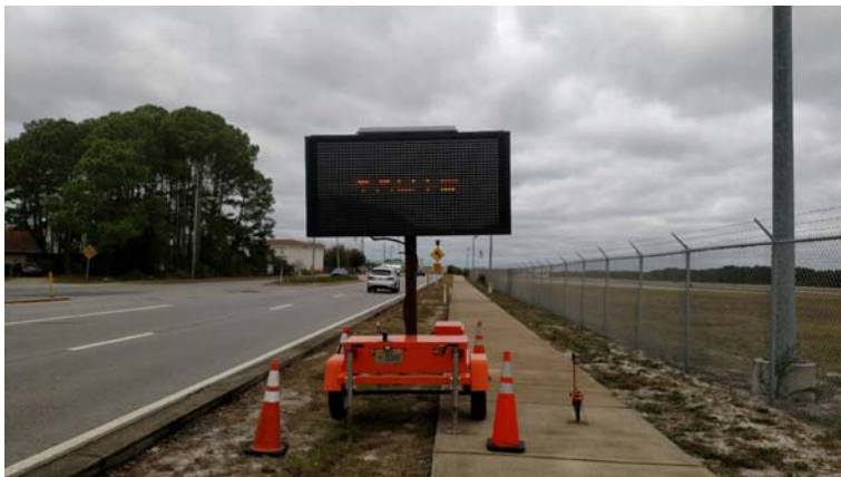
Existing PCMS placed in the westbound shoulder prior to the Airport Road curve warning motorists to "slow down"
