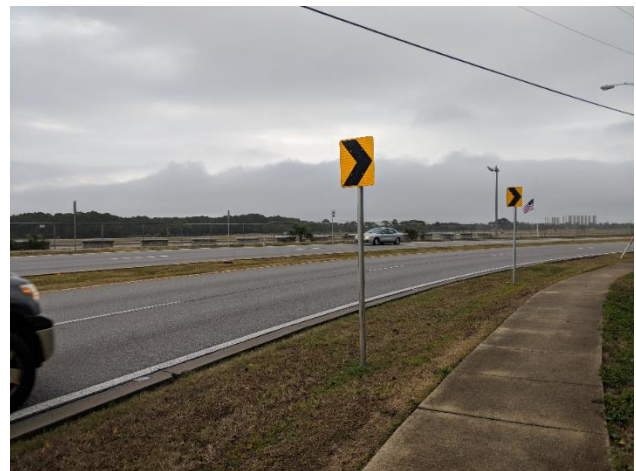
Figure 3 - Inadequate signage and reflectivity
