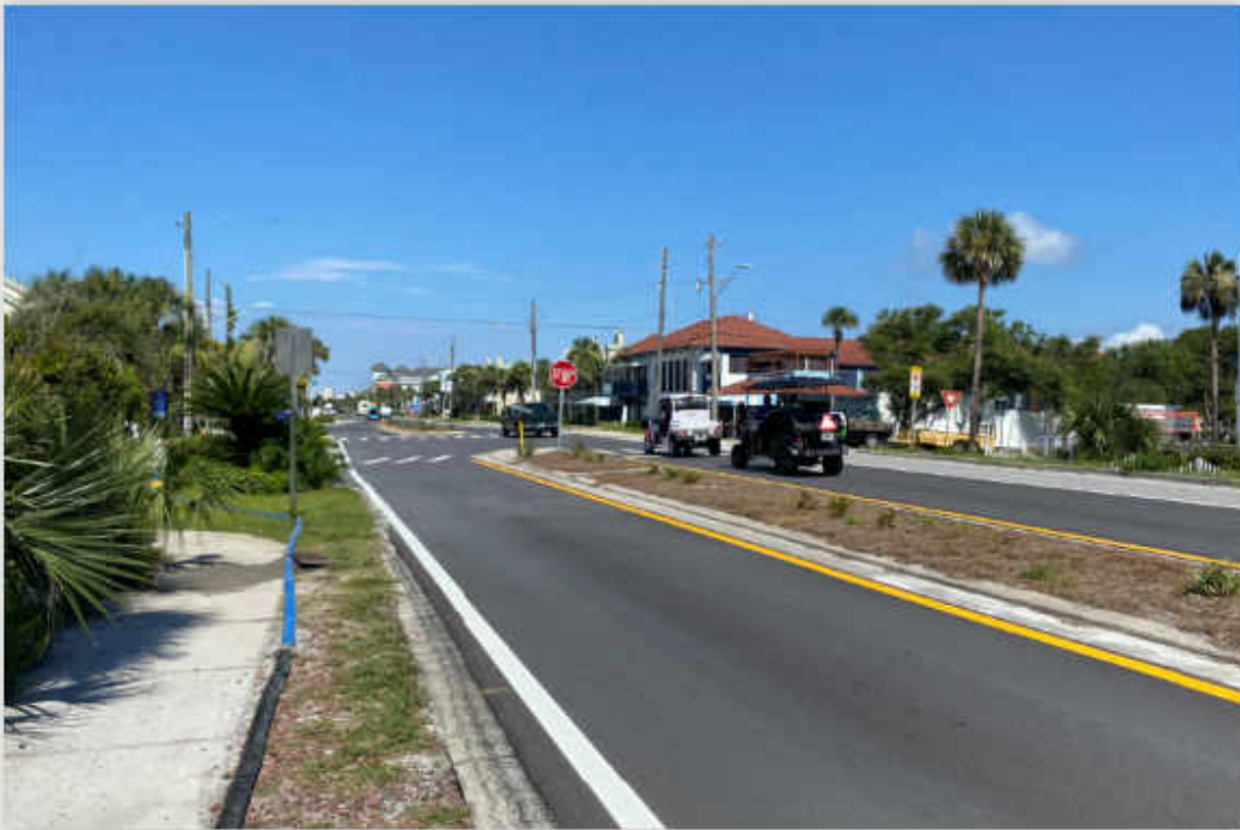
Scenic Highway 98 Viewing West, Subject on Left
