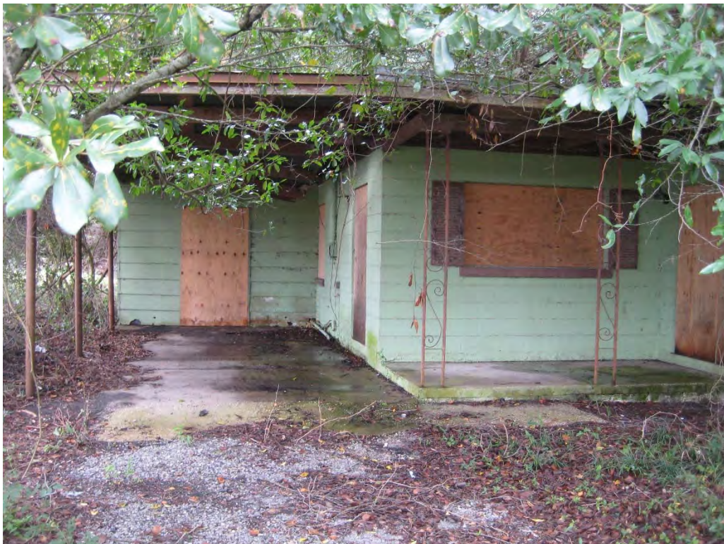
Photo 18 View of residential structure from the west (front)
