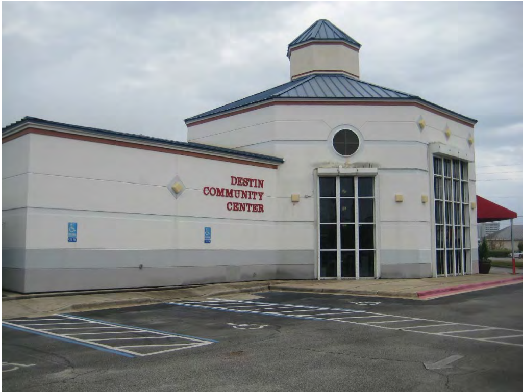
Photo 3 View of east adjacent municipal building
