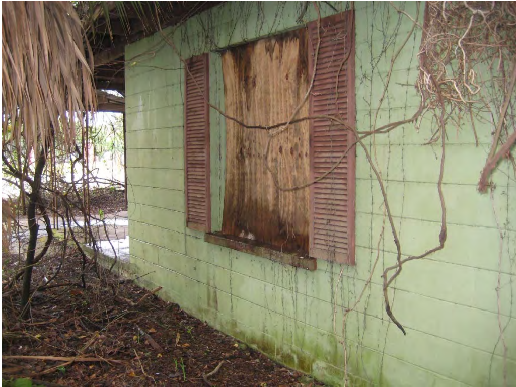
Photo 15 View of residential structure, north elevation
