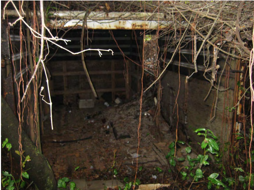
Photo 19 View of storage structure (converted box trailer) from the west
