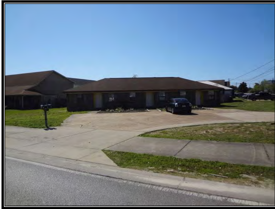
Looking Southeast at the Subject from Legion Drive – Photo #1
