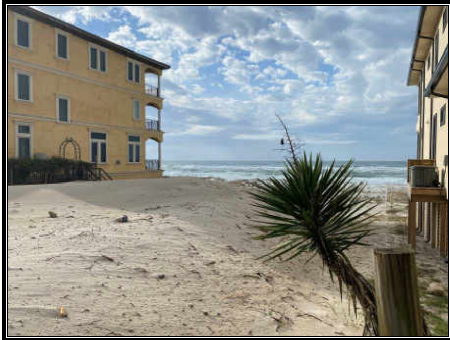
Interior of Subject Site
