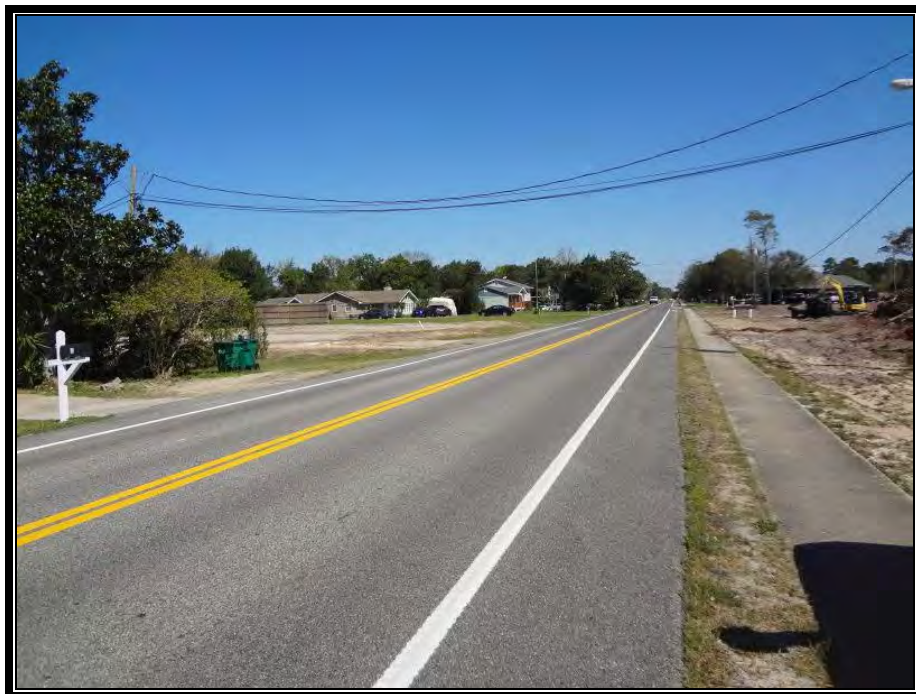
Looking North along Benning Drive – Photo #4
