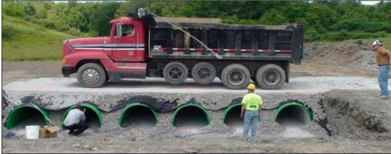
TRITON S-22 INSTALLATION SECTION VIEW
