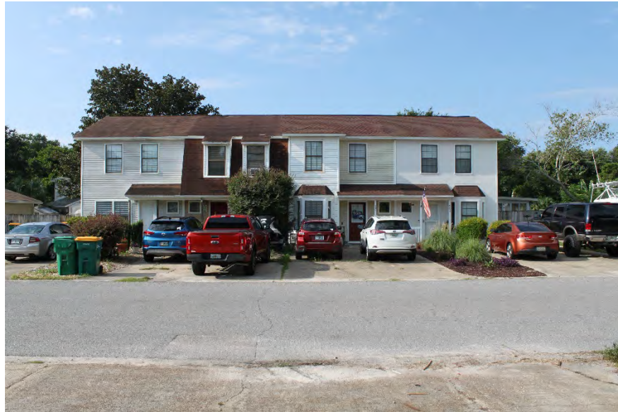
Subject on left side, end unit
