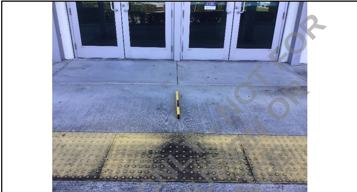
Photo 113: Running slope being obtained at north entrance. Measurement was observed to be 7.4% which meets the requirements.
