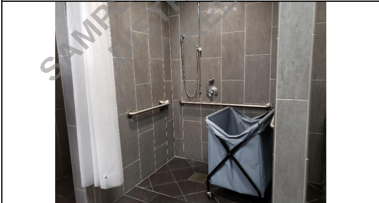
Photo 84: Typical plumbing fixtures in locker room showers
