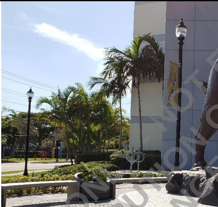
Photo 91: Outside pole mounted lighting.
