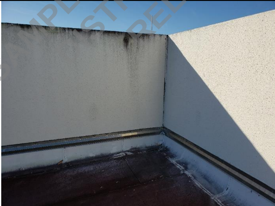
Photo 67: Typical roof membrane termination at parapet wall.
