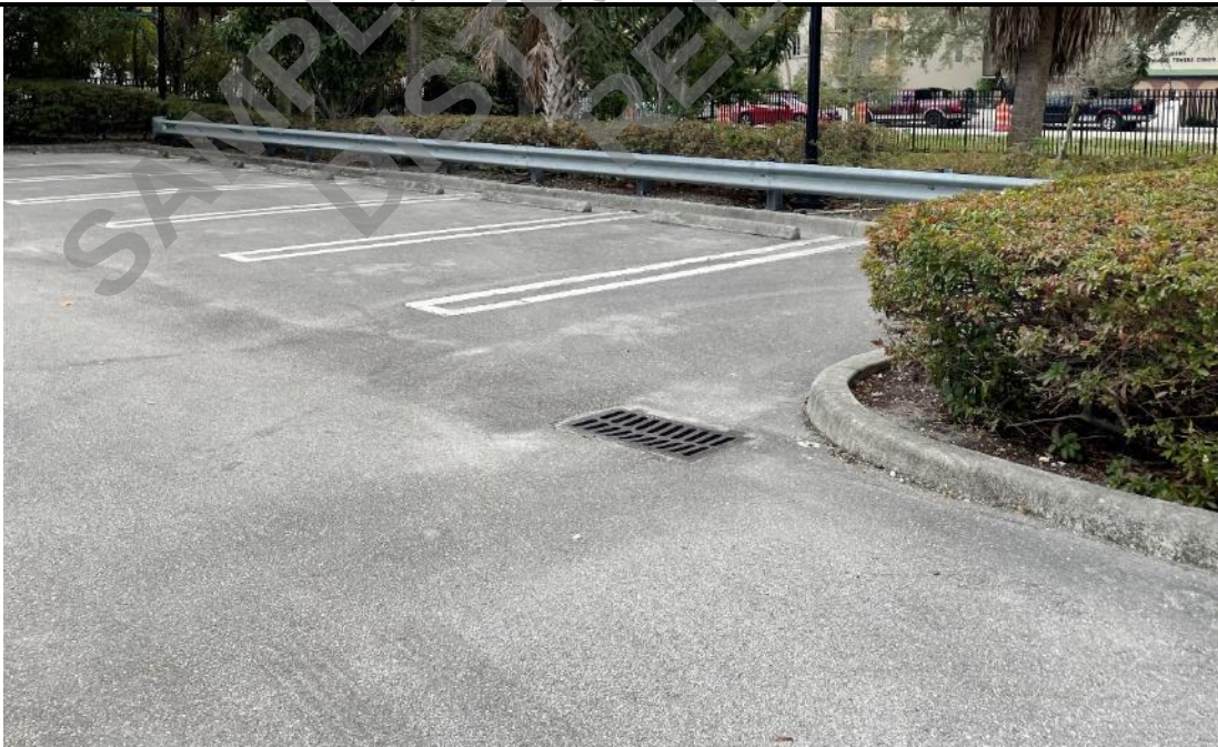
Photo 6: Stormwater drop inlet located at west side parking area.
