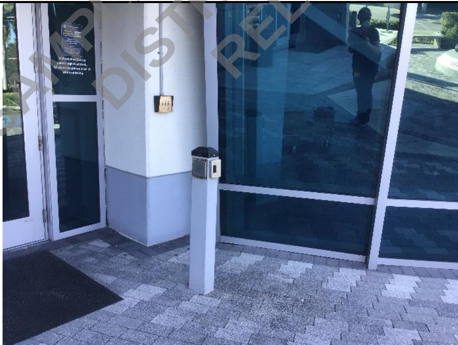
Photo 120: Automatic door opener at east elevation entrance.
