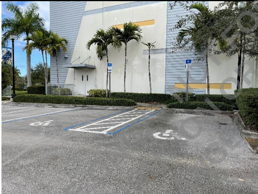
Photo 105: Designated ADA parking spots at west side of building.
