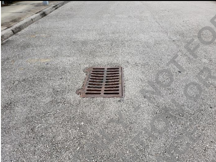
Photo 5: Stormwater drop inlet in drop-off lane.
