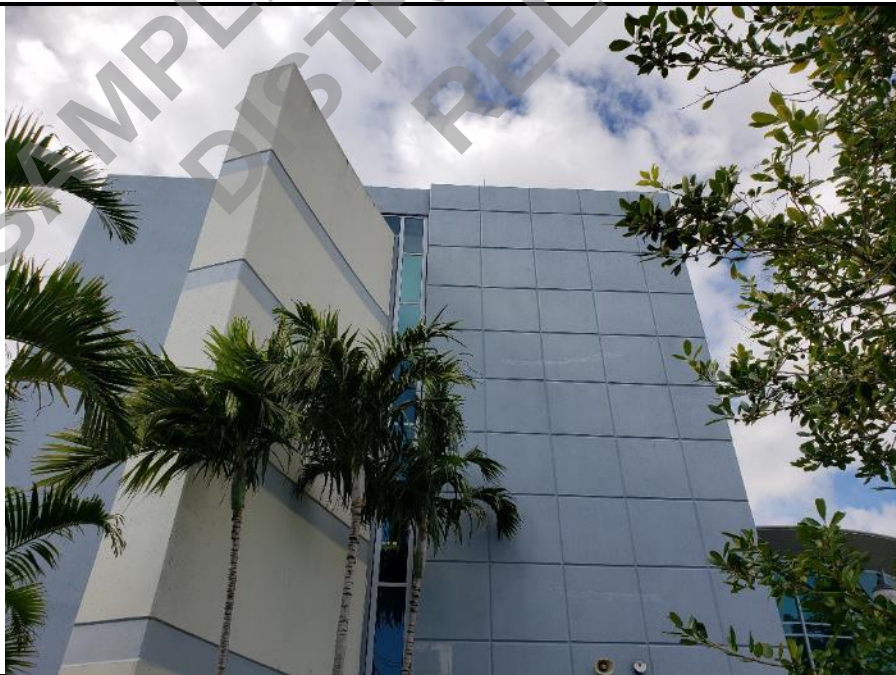
Photo 41: Concrete tilt panels and curtainwall at east elevation.
