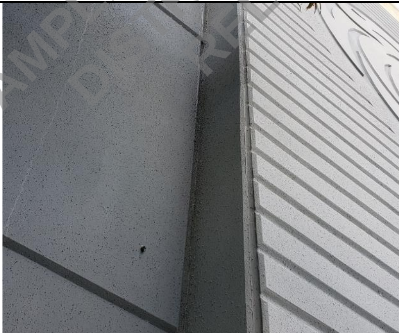
Photo 45: Typical control joint observed for tilt-wall panels.
