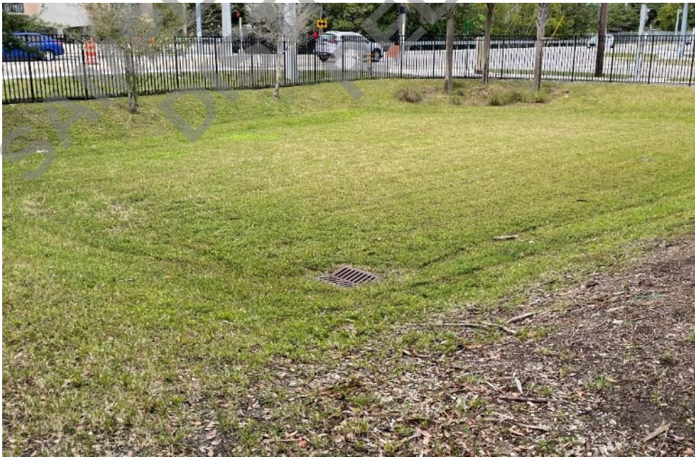
Photo 8: Drainage at detention pond on west side of property.
