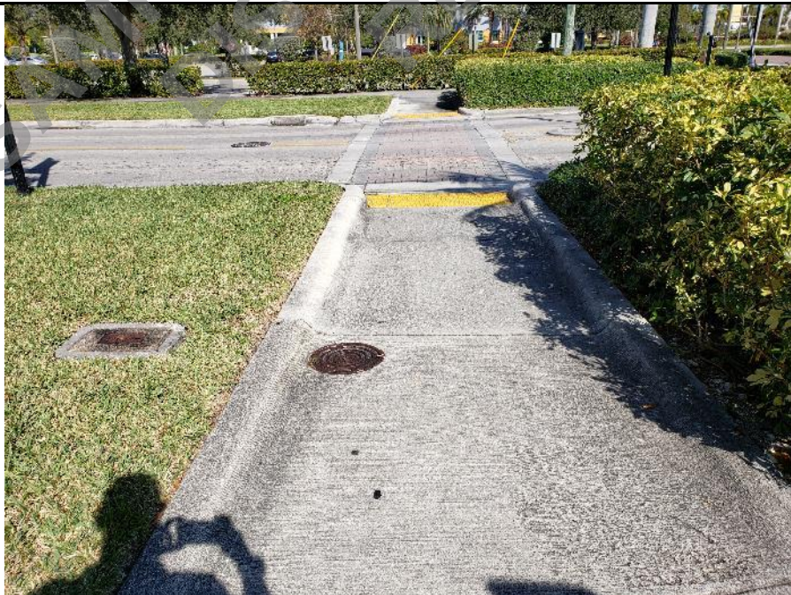
Photo 106: Marked cross walks leading to building
