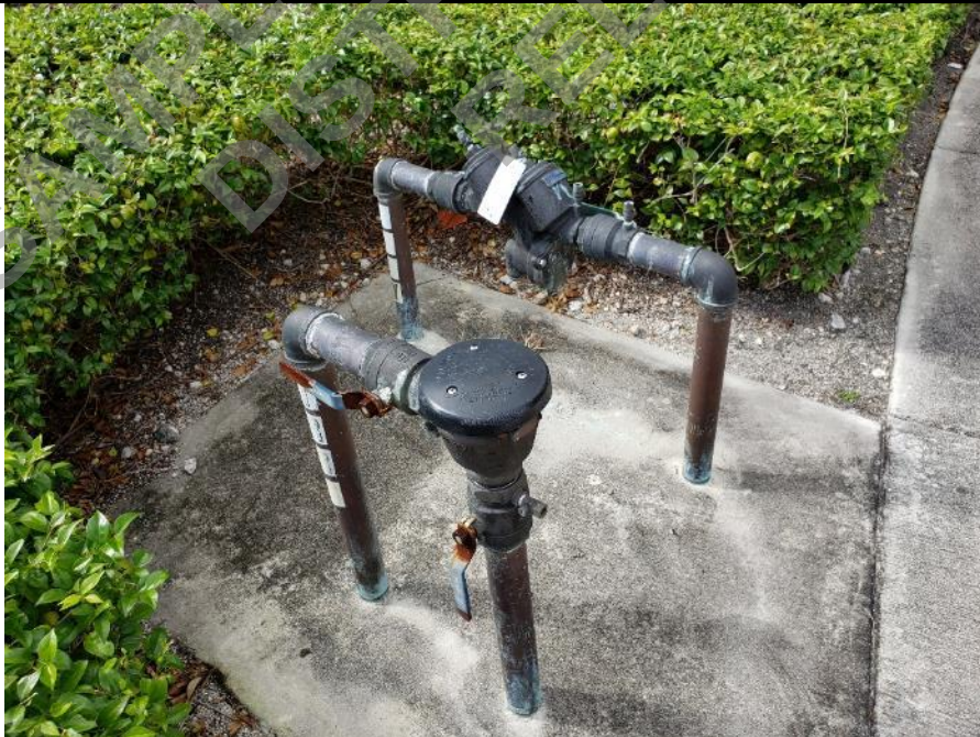
Photo 33: Water service near main north east courtyard.
