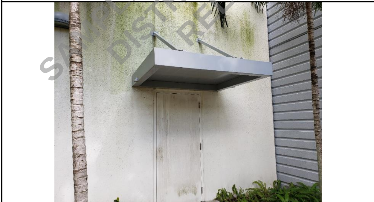
Photo 55: Typical awning at south elevation.
