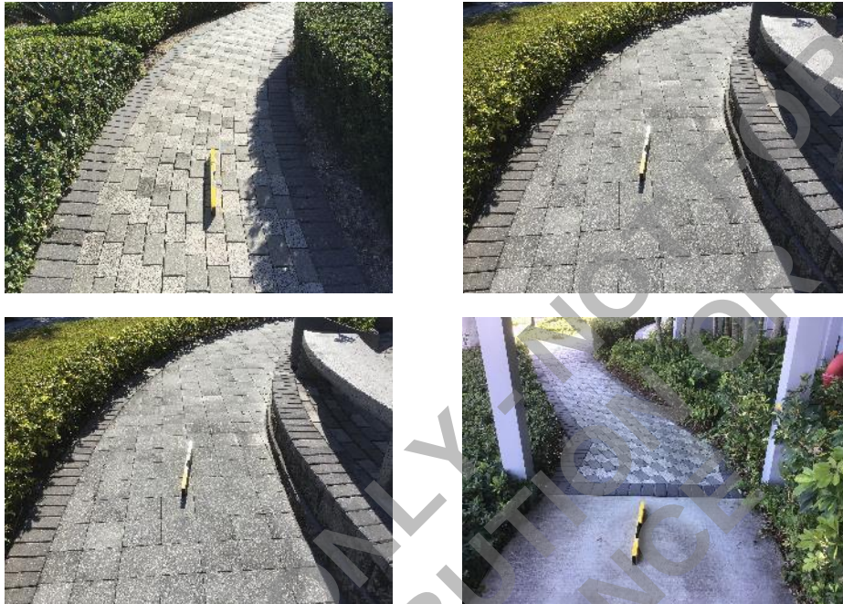
Photo 117: Slope measurements were obtained along the accessible route at the east entrance to the building. All measurements obtained were within acceptable thresholds, under 5% for running slope and 2.08% for cross slope.
