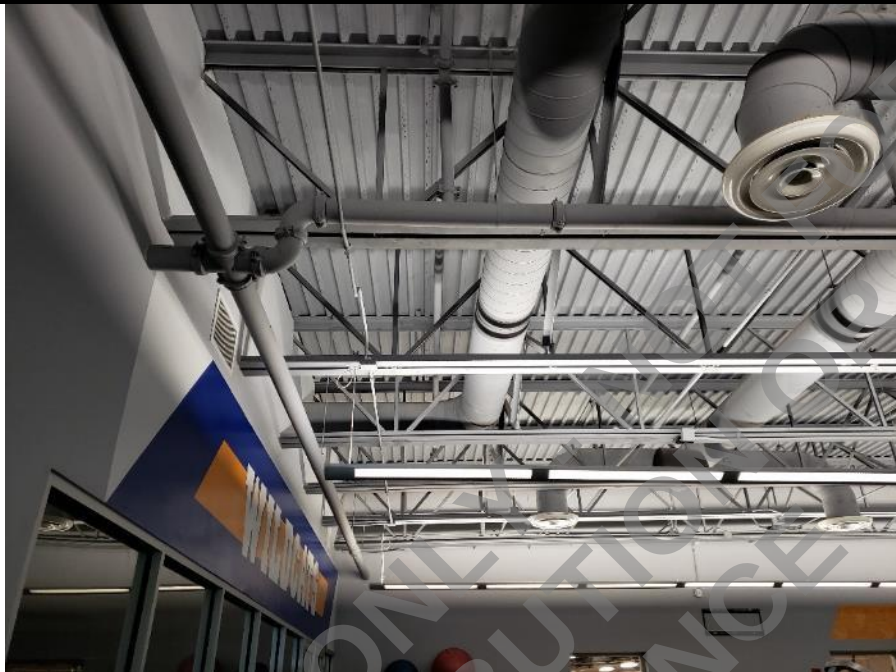
Photo 38: Typical framing consisting of steel joists supporting a corrugated metal deck.
