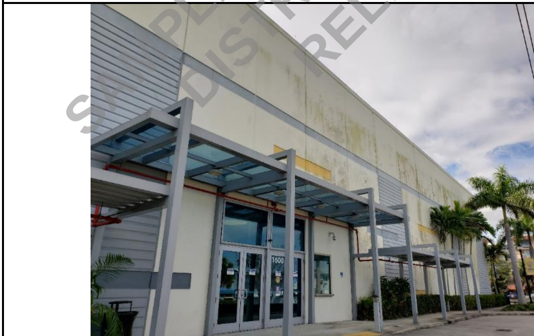
Photo 35: Typical exterior view of building elevation, north side.
