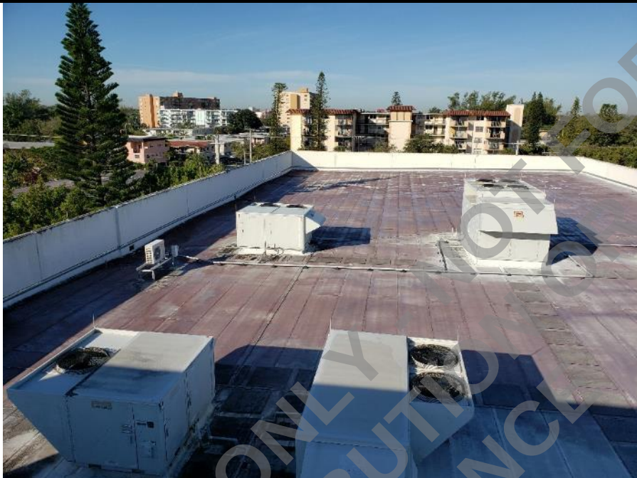
Photo 60: Roof system overview over basketball court.
