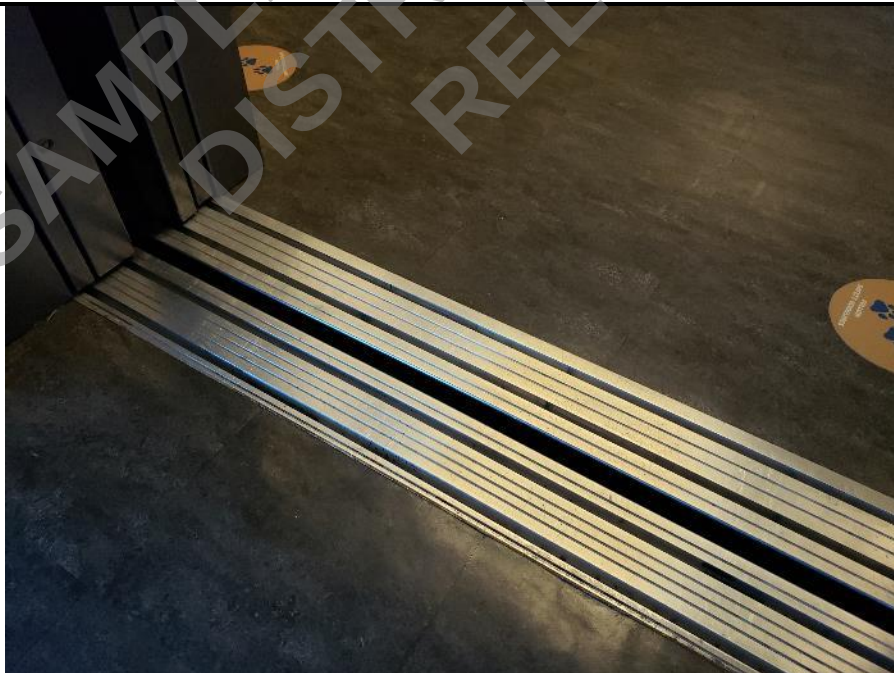
Photo 112: Threshold at elevator cab.
