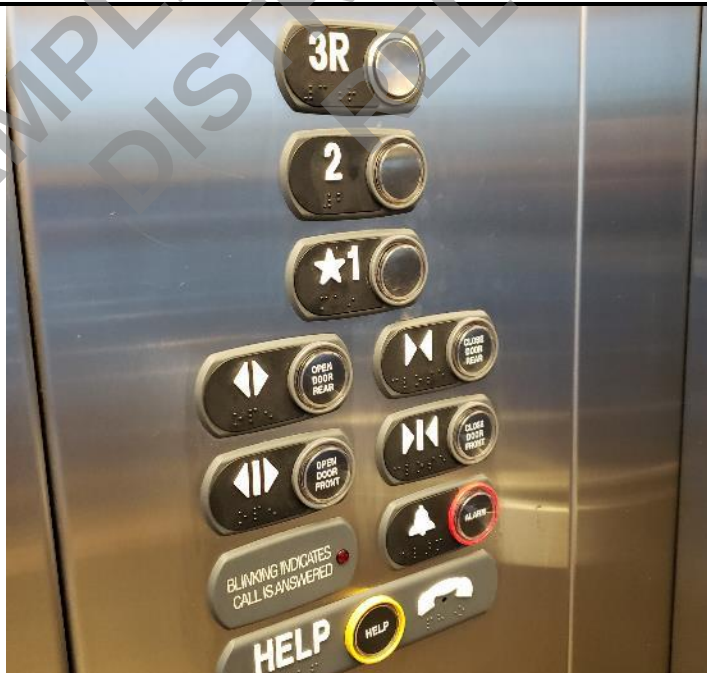
Photo 110: Braille markings on elevator controls.
