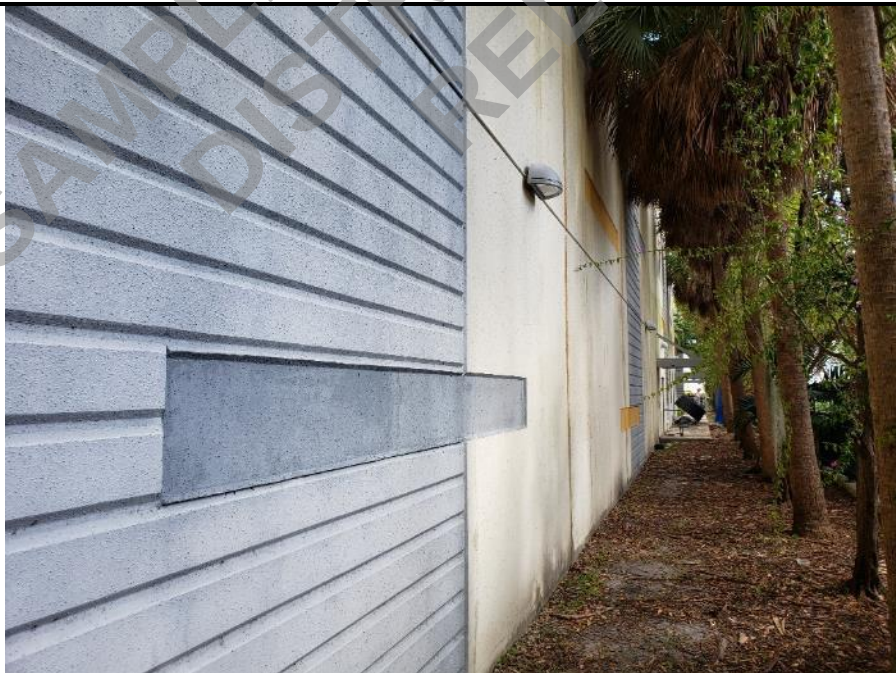
Photo 37: View of south elevation.
