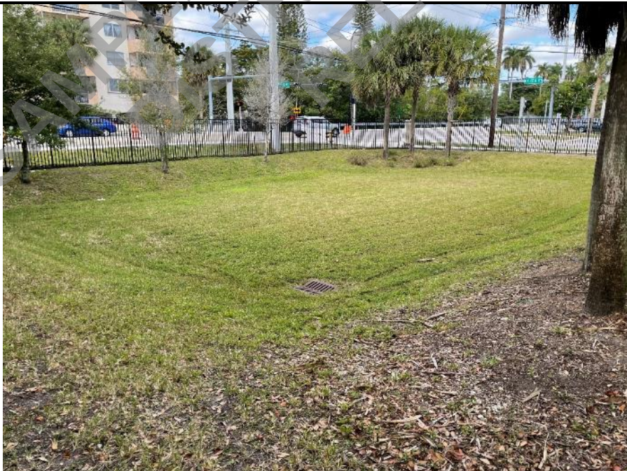
Photo 26: Detention pond on west side of property.
