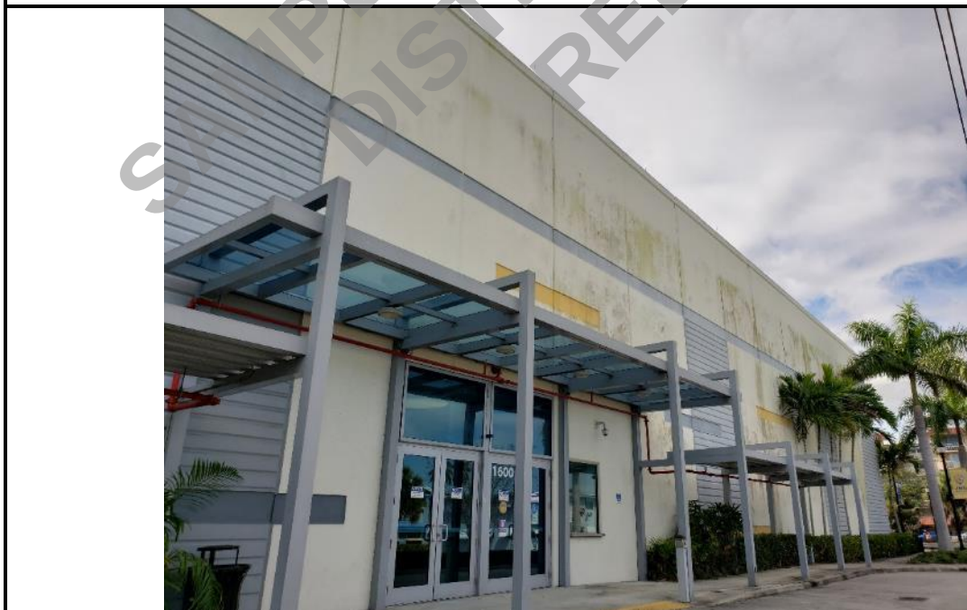
Photo 53: Awning over north entrance extending along sidewalk.
