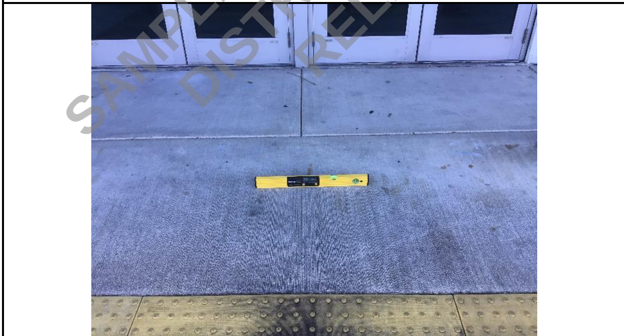
Photo 114: Cross slope measurement being obtained at north entrance ramp. Measurement was observed to be 0.2% which meets the requirements.
