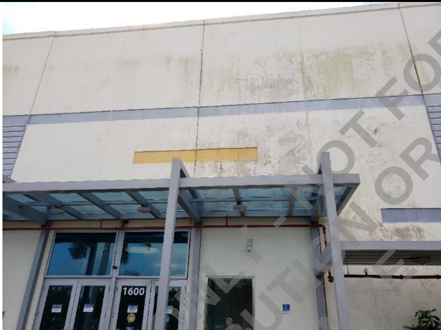
Photo 36: Concrete tilt-up wall panels and aluminum framed entrances and storefronts make up the exterior elevations of the buildings.
