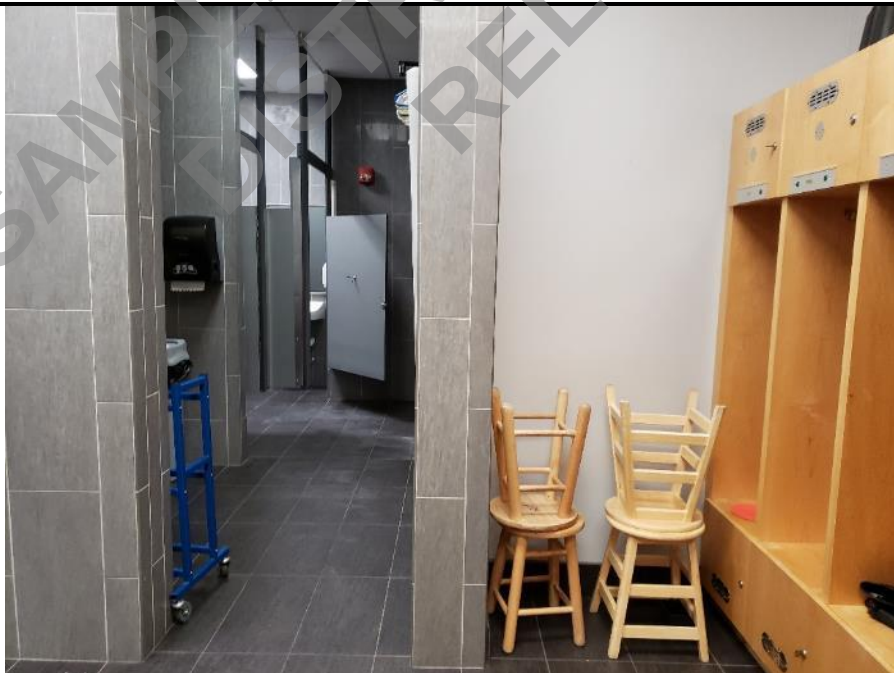
Photo 74: Typical interior finishes in locker rooms.
