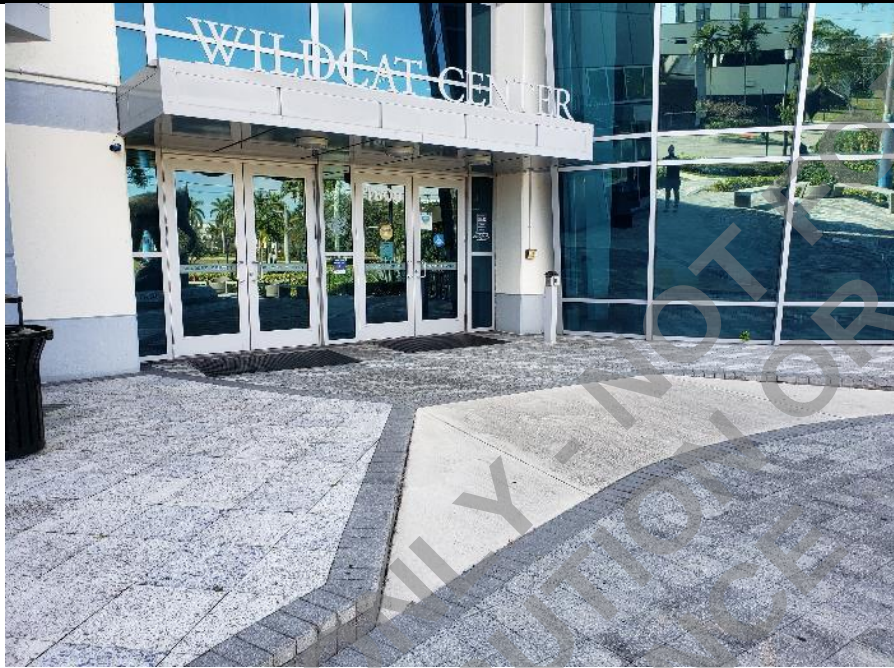
Photo 111: Main entrance ramp with ADA signage and automatic door opener.
