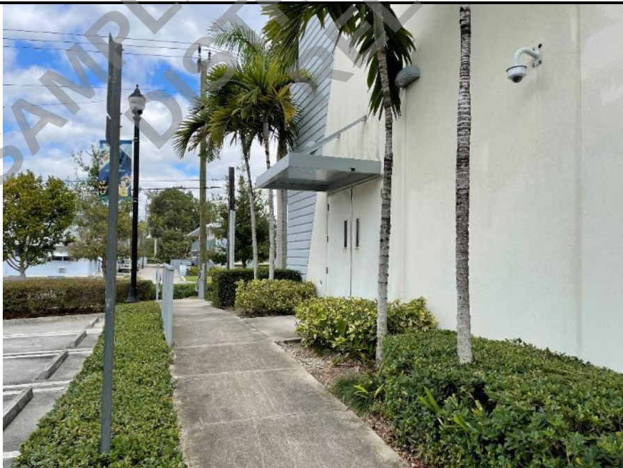
Photo 18: Sidewalk at west building perimeter.
