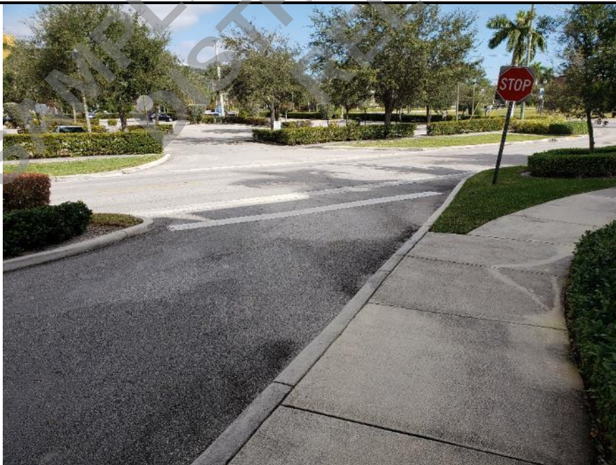
Photo 16: Typical curbing at drop off lane.
