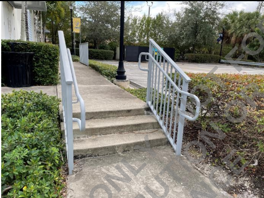
Photo 17: Sidewalk and stairs at west side of building.
