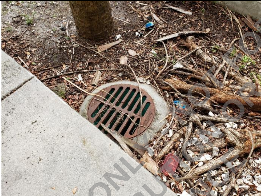
Photo 7: Sewer inlet at south side property line.
