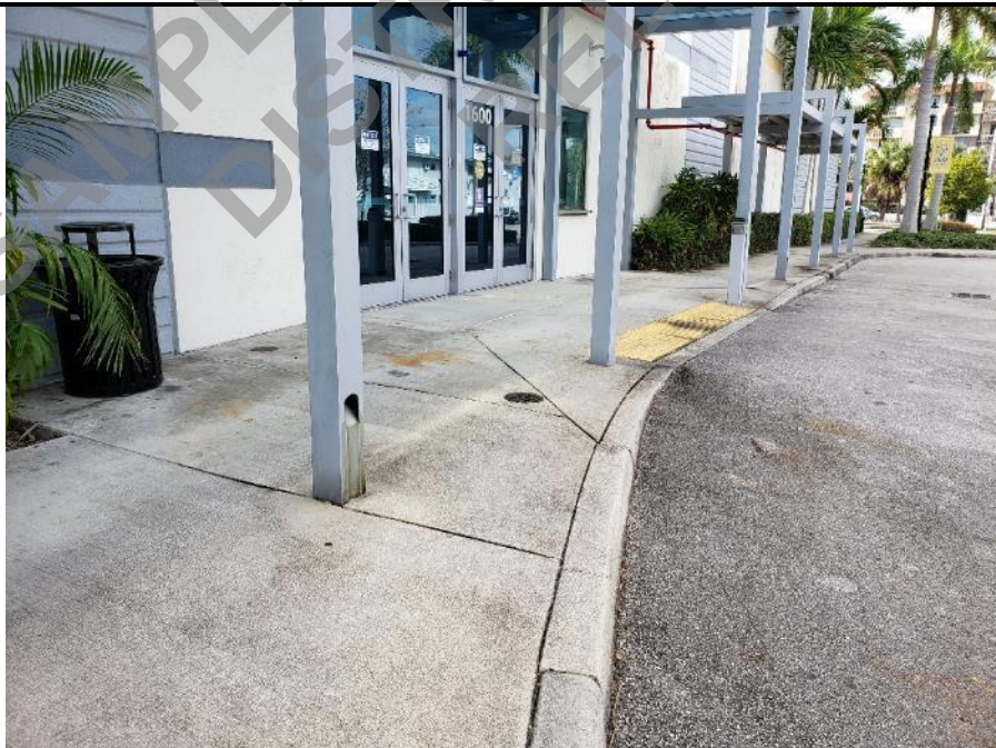
Photo 20: Flatwork at north gym entrance.
