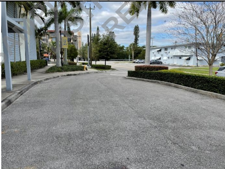
Photo 14: Asphalt drop off lane on north side.
