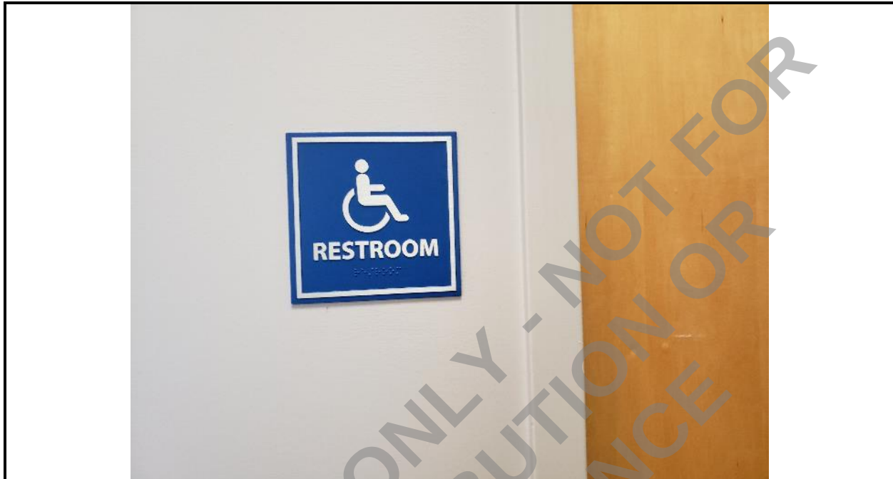
Photo 107: ADA restroom signage with Braille Markings
