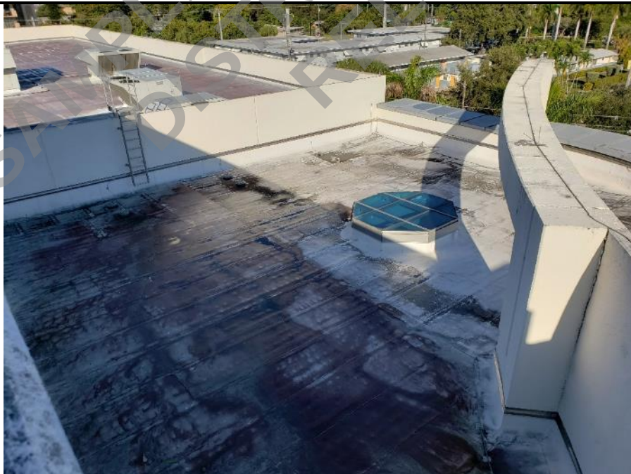
Photo 59: Roof system overview over lobby entrance.
