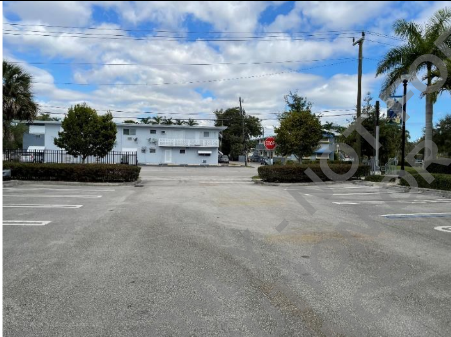
Photo 13: Asphalt parking on west parking lot.
