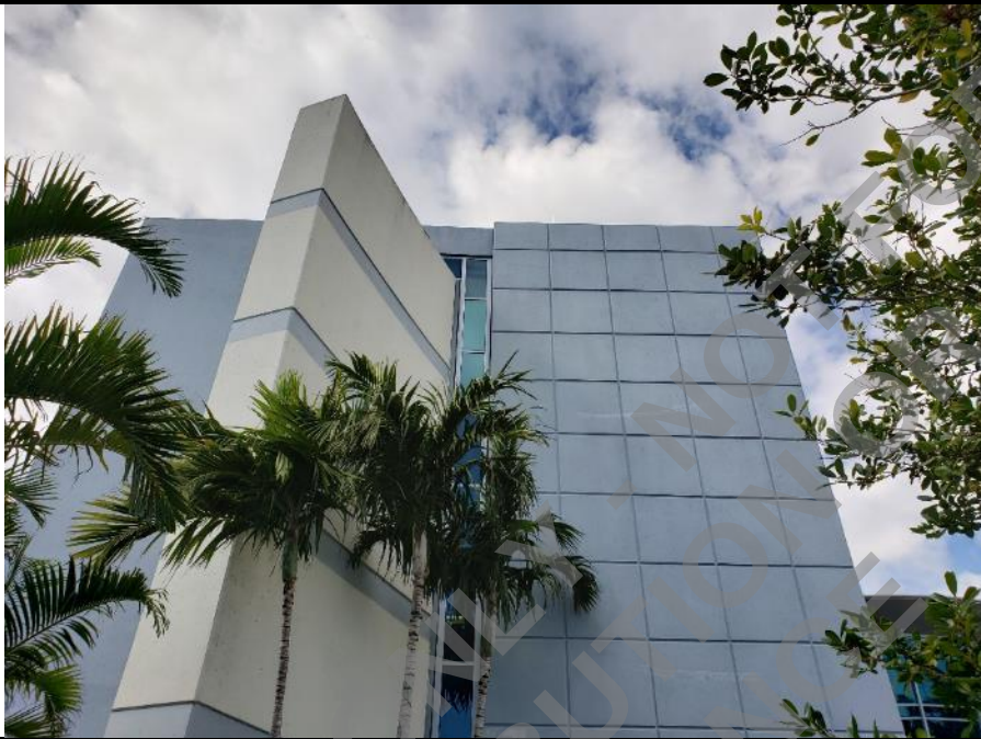
Photo 48: Curtainwall system at east elevation.
