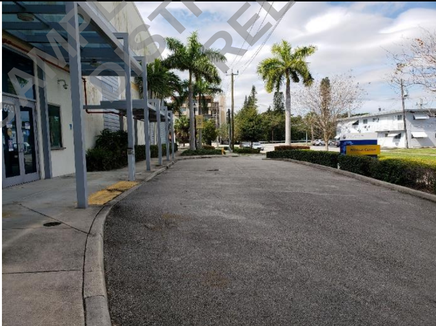
Photo 10: View of pedestrian and vehicular access from NE 126 th Street.
