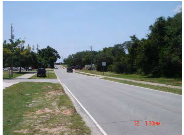
Street View Southerly
