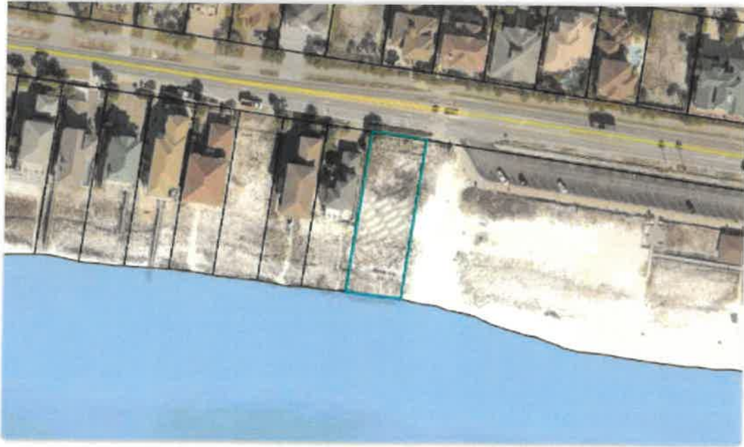
Aerial Photograph of Site
